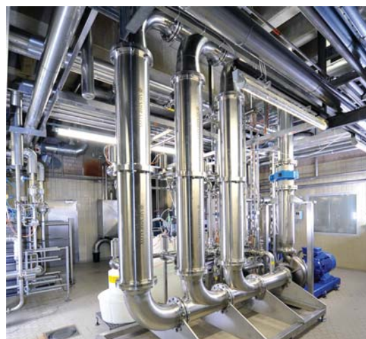
Keraflux-TFF System 3 x 2 HCB Membranes
